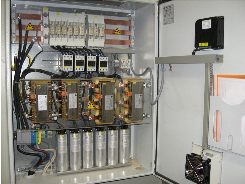
Figure 12. Example of a power factor correction unit used for plant-wide power factor correction. Notice the six capacitors (two per phase) located at the bottom of the unit.
