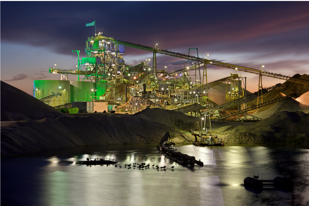
Figure 1. Large industrial plants containing motors and other reactive loads in constant or near constant operation (such as the large conveyors in the mining plant in the above figure) greatly benefit from power factor correction.
