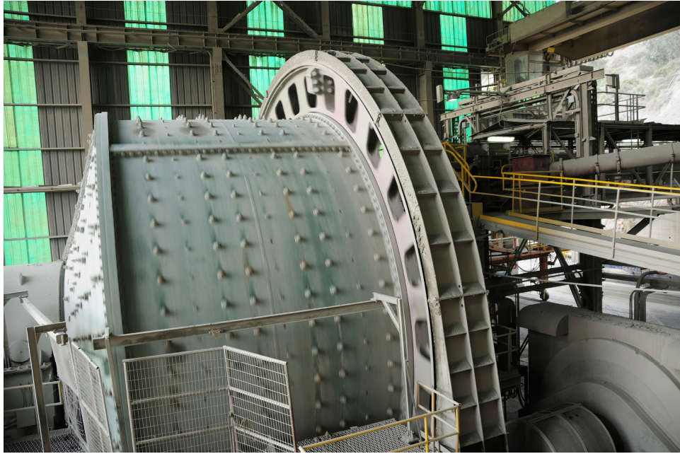
Figure 10. Any induction motor driving a large load such as the ball mill shown above requires a substantial amount of reactive power to operate. Using distributed power factor correction prevents the large reactive power requirement of the motor from affecting the power factor of the industrial application.
